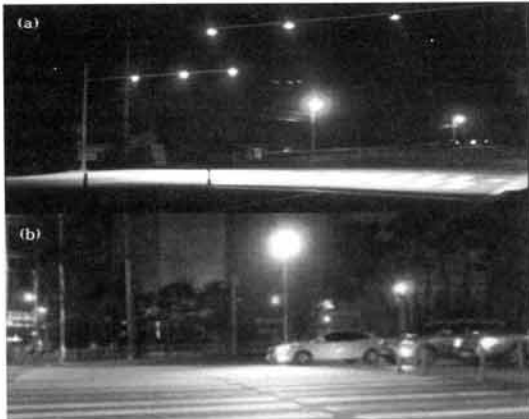
Fig. 1. Installations of LED crosswalk (a) division of LED crosswalk, (b) a single of LED crosswalk.
