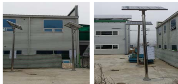
Fig. 9. Installation of solar LED street lamp to compare the power generation efficiency.
