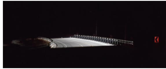
Fig. 1. Character of low-deck lighting road.
