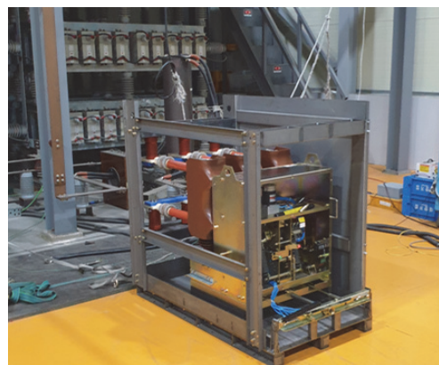
Fig. 2. Vacuum circuit breaker for testing current conditioning.
