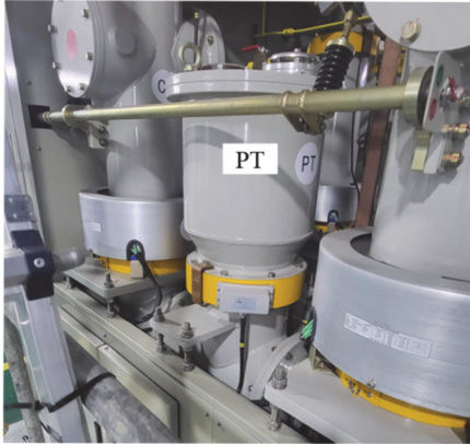
Fig. 1. Application of tank type PT in GIS.
